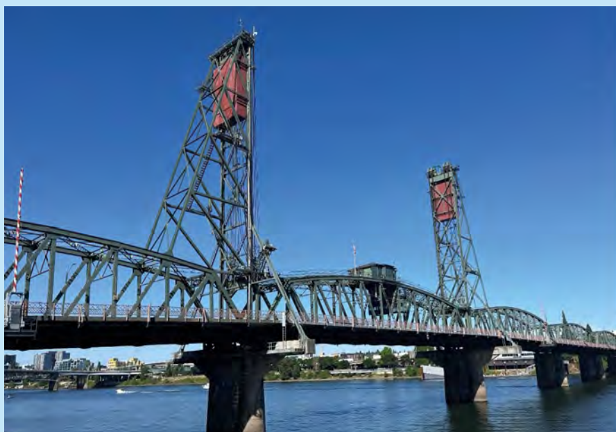
Hawthorne Bridge, lyftbro i Portland. Foto: Charlotta Nordlöf
