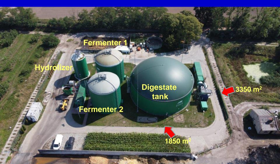
The actual state: linear (24 h/day) production of electric energy and heat (cold production for fruits freezer and ORC system planned probably since 2025)
