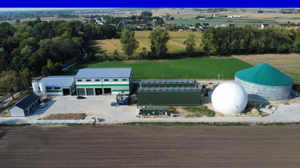
Biogas plant in Przybroda farm: 0.5 MW → 1 MW (2024) One of the most advanced biogas plant in the World Surface for biogas plant: 1850 m<sup>2</sup>, Total surface of parcel: 3350 m<sup>2</sup> Substrates: manure from 200 cows, agricultural biomass
