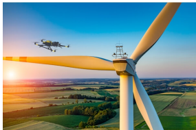
Wind turbine inspection
