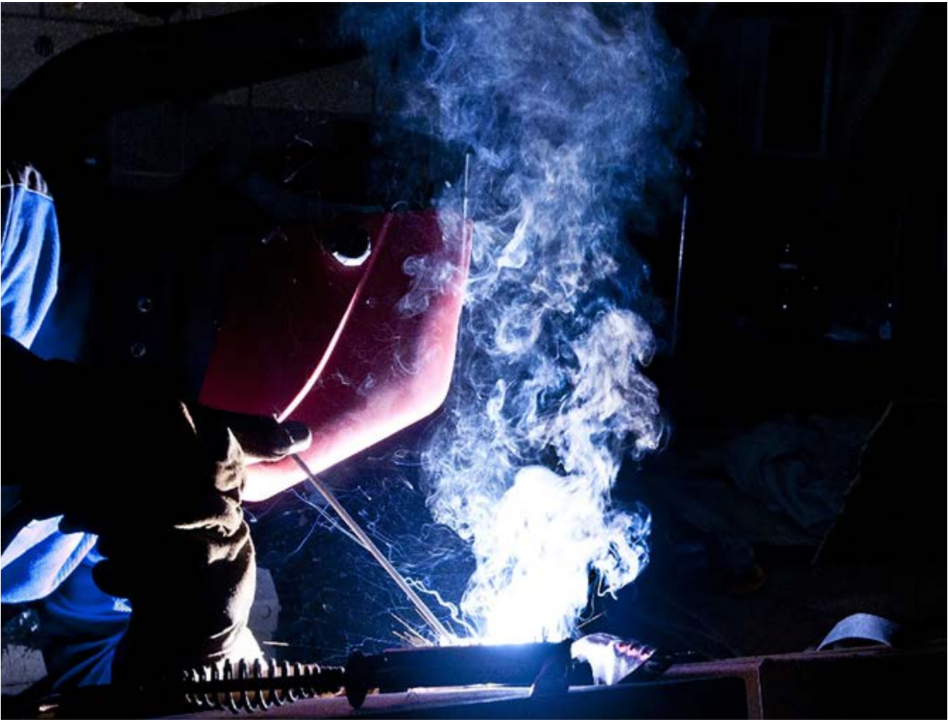
Welding in progress.
