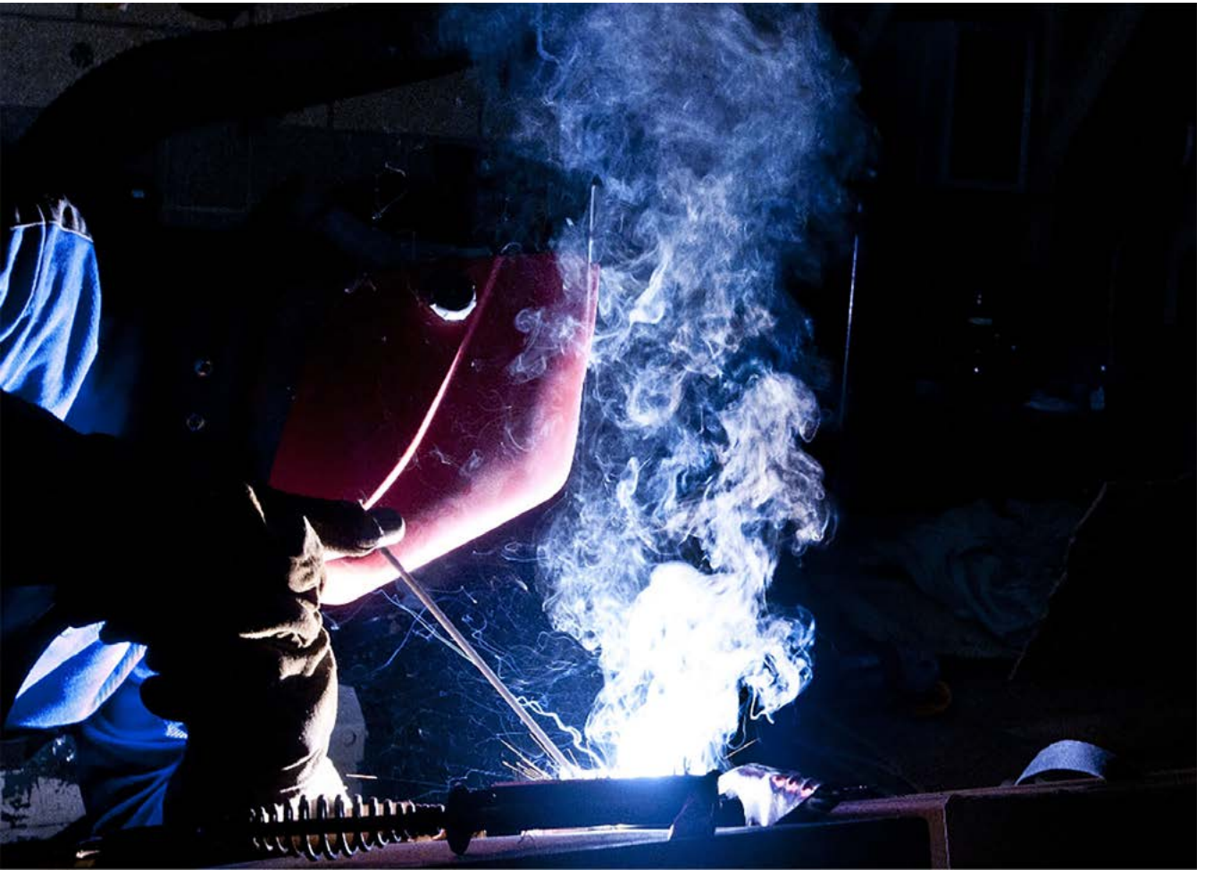
Welding in progress.
