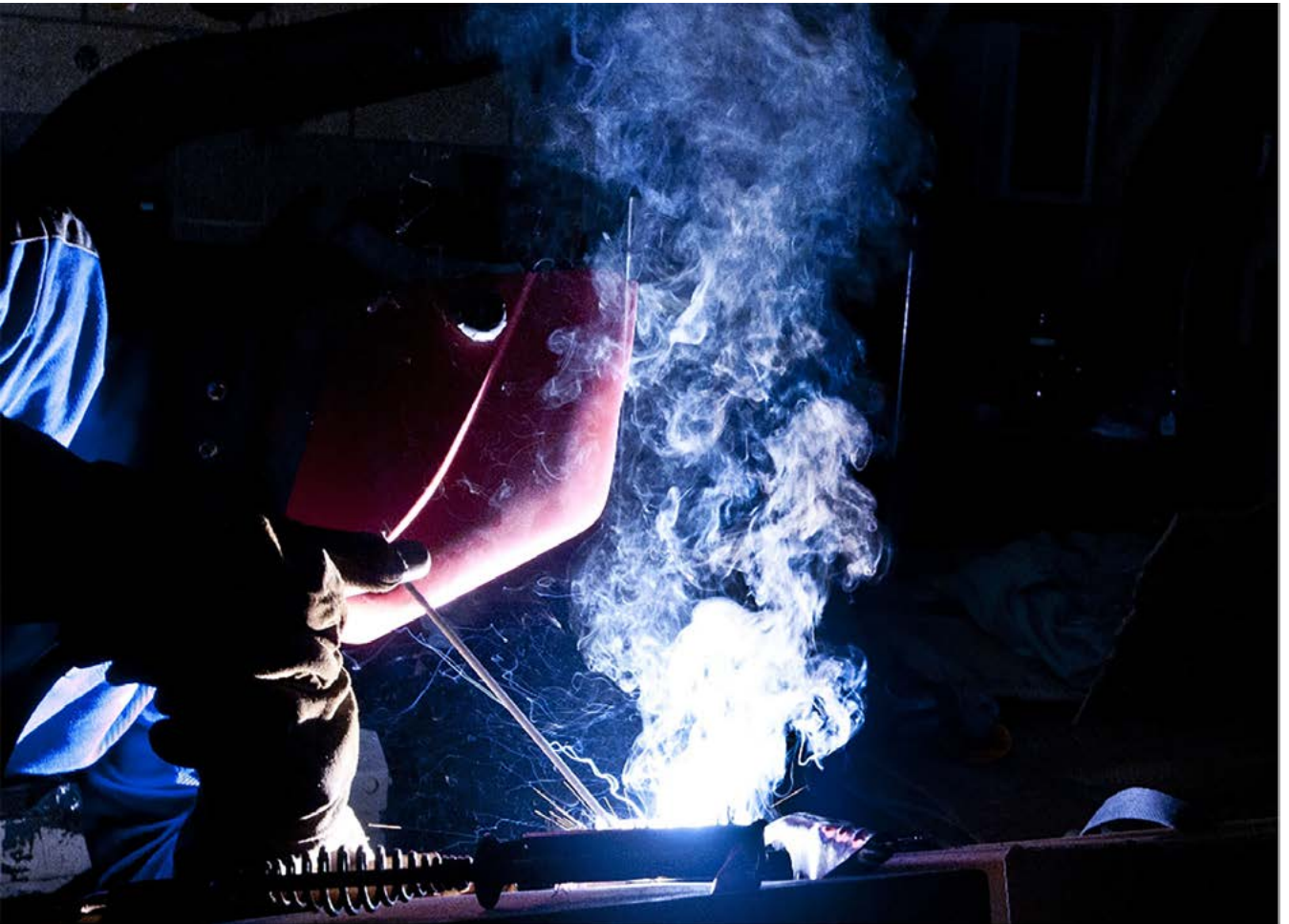
Welding in progress.
