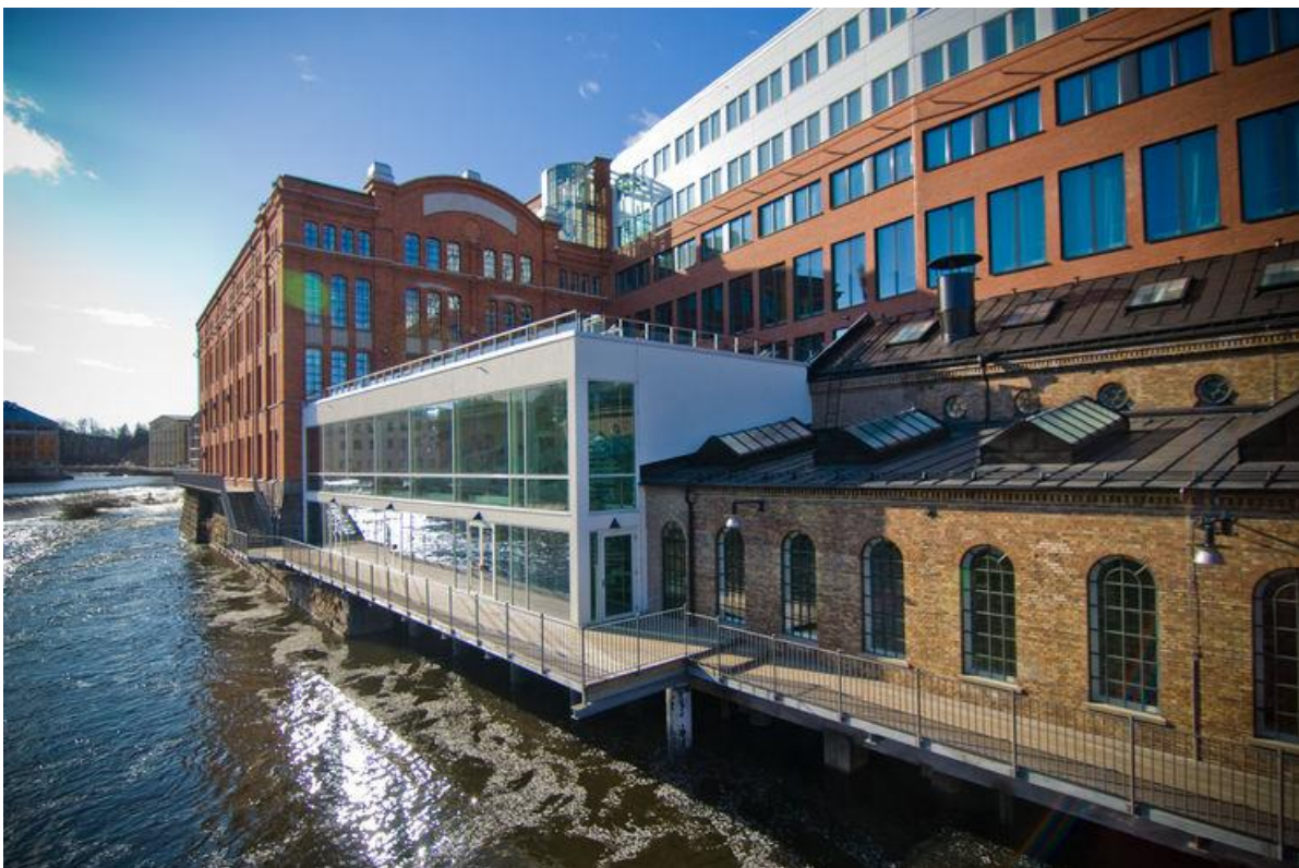
Kåkenhus, Campus Norrköping. Peter Modin
